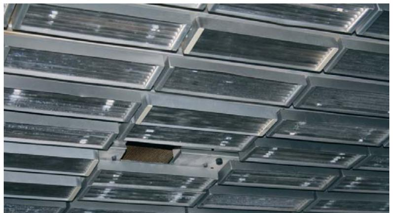
Picture 1: Heating field consisting of emitters, arranged in columns and rows. One heating field has been removed for the field of view of the camera
